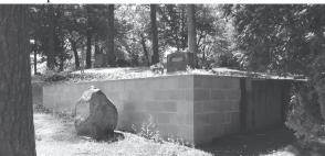
The two retaining walls that were falling on the west side of the cemetery were replaced with new reinforced block retaining walls. After removing the old walls it was found they were not installed with any reinforcement many, many years ago when they were put up. The new walls should look great for many years to come. Thank you to MCU Construction. See picture below.
